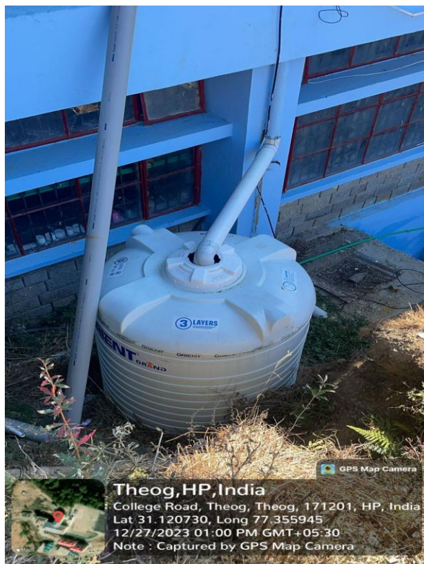
Rainwater harvesting Tank and its connectivity to Botanical glass house and Toilet
